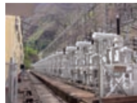
Installation of substations
