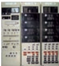
Digital-type monitoring and control devices
