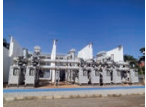
Queensway Substation at completion
