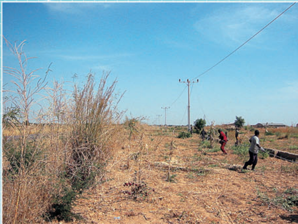
33kV Transmission Line
