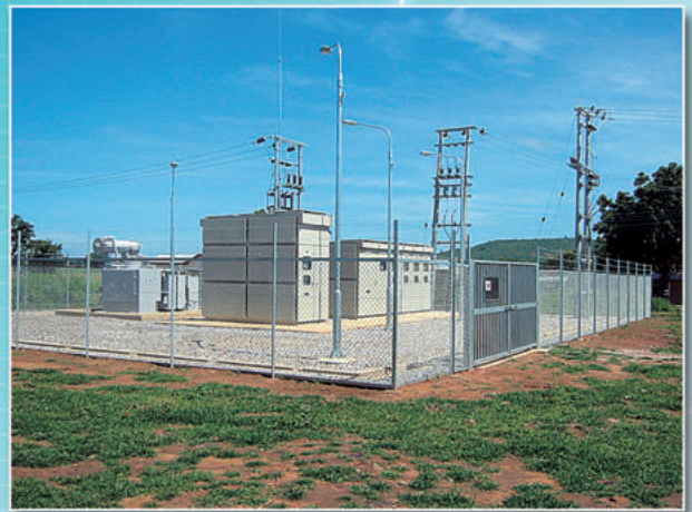
Kalshingi Substation 33/11kV 1000kVA
