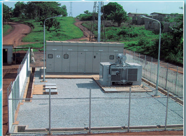
Bibiani Booster Station 5000kVA Booster & 33kV Switchgear
