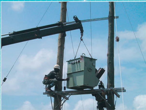
24 units of 33kV 200kVA Distribution Transformer
