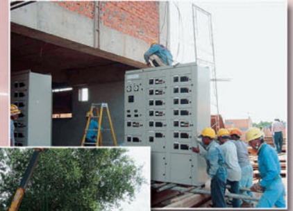
▲ Switchgear Installation
