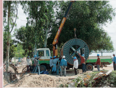
◀ 22kV Cable Installation for Distribution
