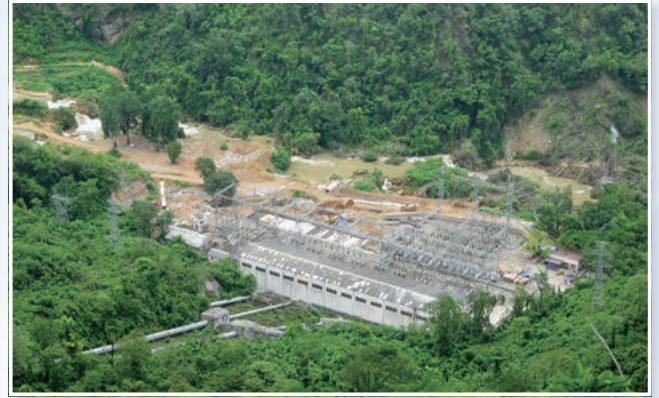
Overall view of the Power Plant
