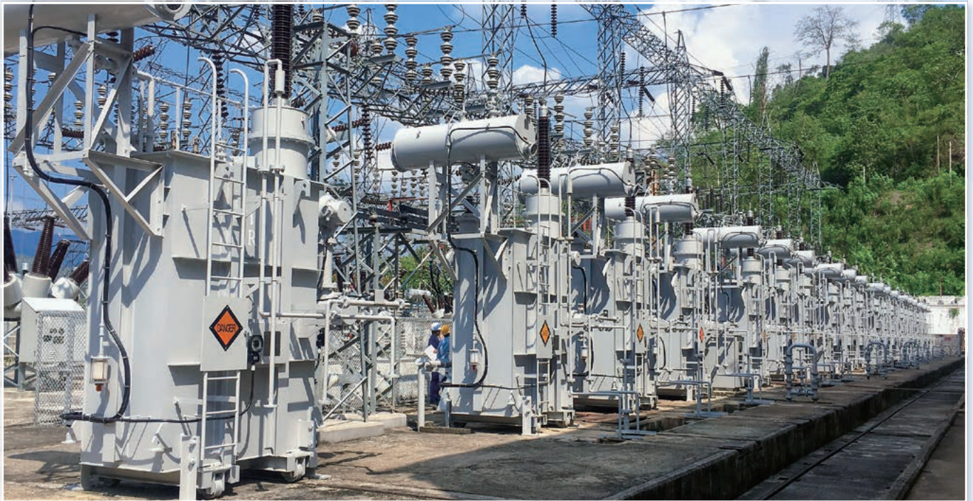
11/132kV Main Transformer
