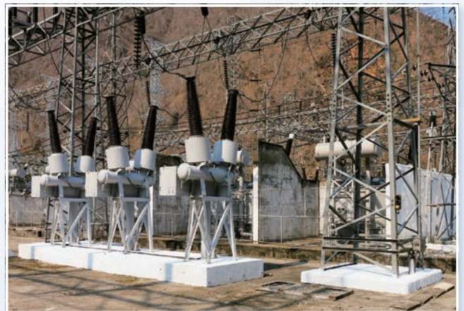
Gas Circuit Breakers
