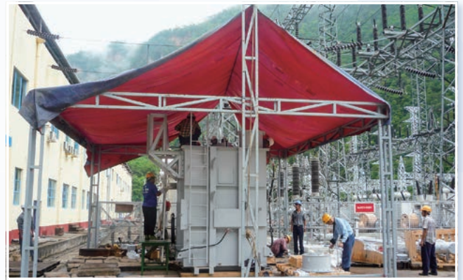
Assembling of Main Transformer
