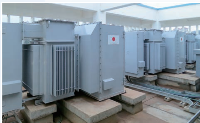
Station Service Transformers
