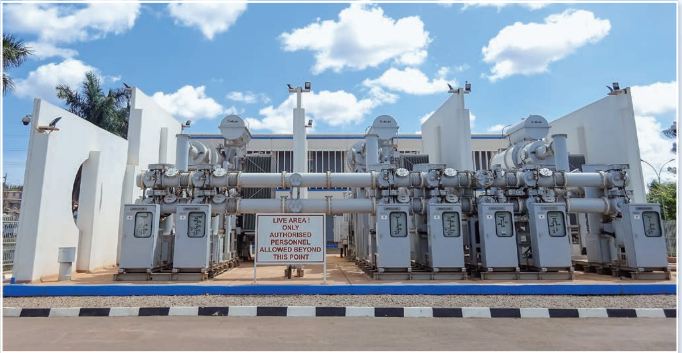
132kV GIS & Main Transformer
