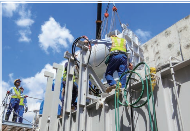
Assembling of Main Transformer
