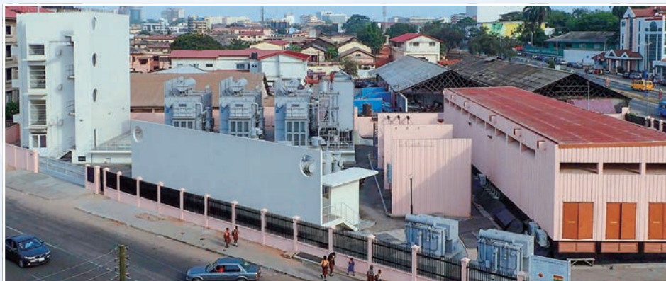
Panoramic View of Substation
