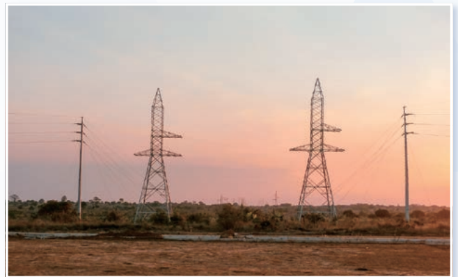
Power Transmission Tower (Namialo)
