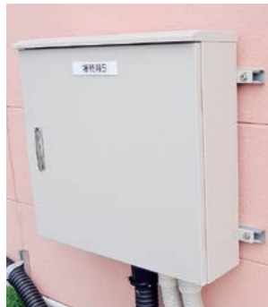
接続箱▶ Junction box
