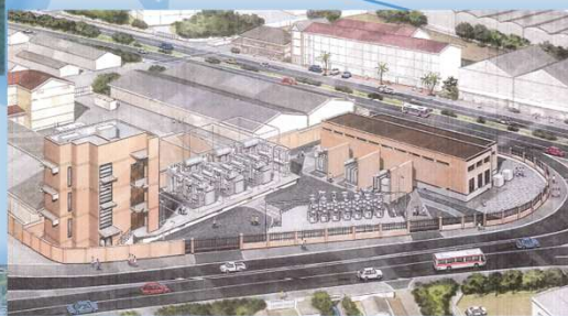
Ghana Project, on-going 2018 (161/34.5kV 125MVA x 3 GIS)
