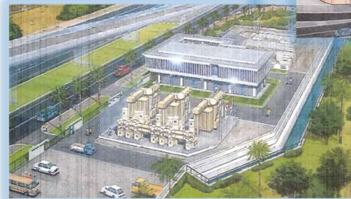
Uganda Project, on-going 2017 (132/33kV 40MVA x 3 GIS)
