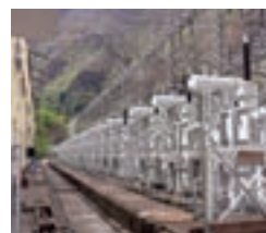
Installation of substations
