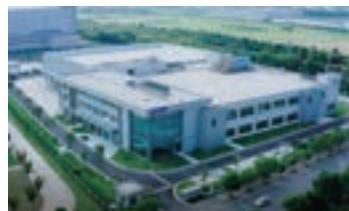
Panorama of the new factory
