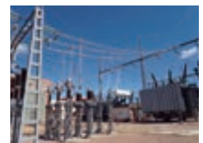
Receiving and transforming substation construction
