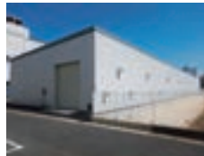
Exterior of the new metal plating factory
