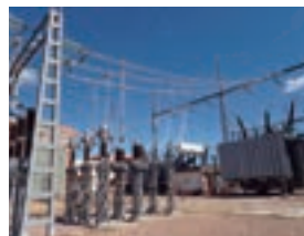
Receiving and transforming substation construction
