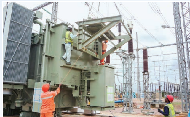
Installation and assembly work
