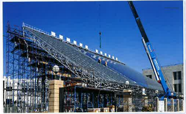
Installation of PV modules
