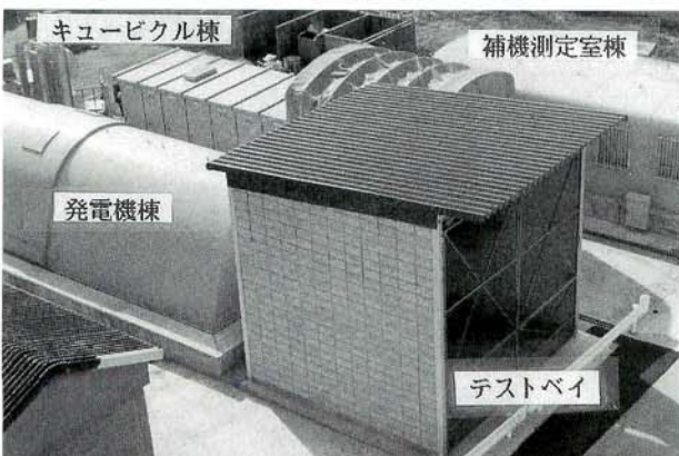
図1 / 短絡試験設備全景 Fig. 1/View of short-circuit testing equipment
